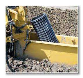
Installation: Installation of DWP is easier because it is easier to handle than traditional materials. For example, 12" DWP weighs 3.4 lbs per foot compared to 10.5 lbs for corrugated metal and 79 lbs for concrete. In some cases this means you can use smaller equipment. DWP can be coupled together with split couplers or snap couplers. 12", 15", 18", 21" and 24". All sizes of dual wall pipe are available with bell ends.
